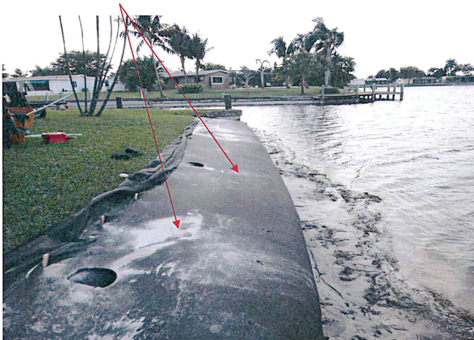
Main Geo-Tube installed and pumped with sand from lake bottom
