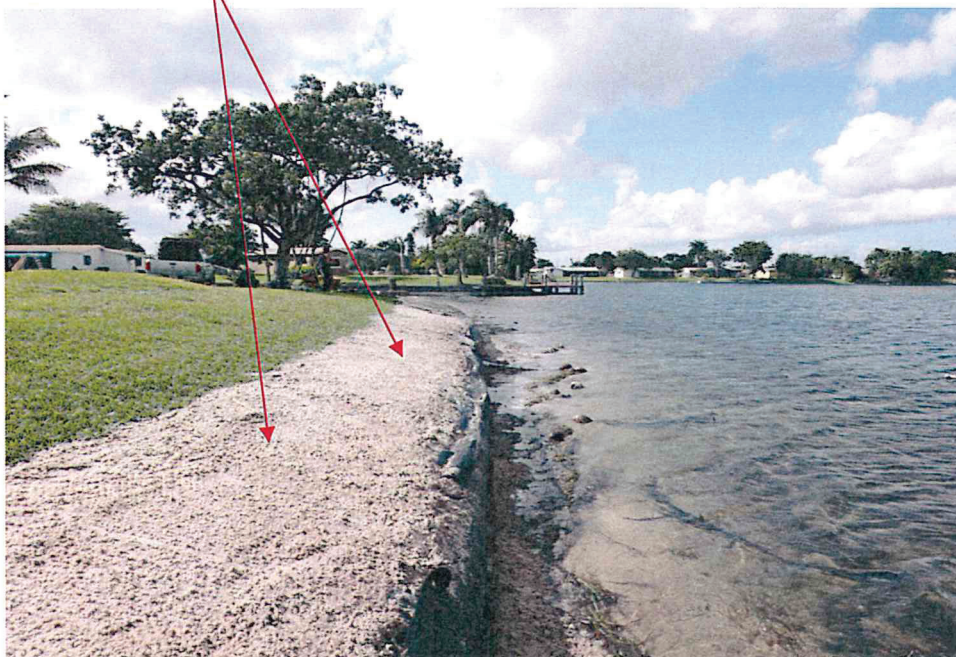
Sand installed over Geo-Tubes and graded to proper slope
