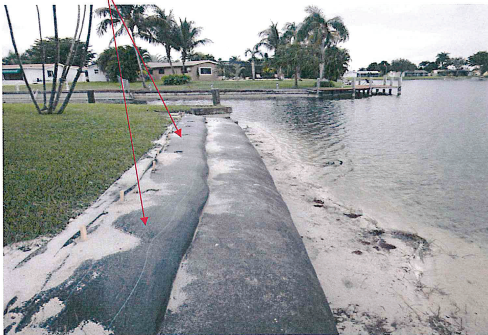
Sand installed over Geo-Tubes and graded to proper slope
