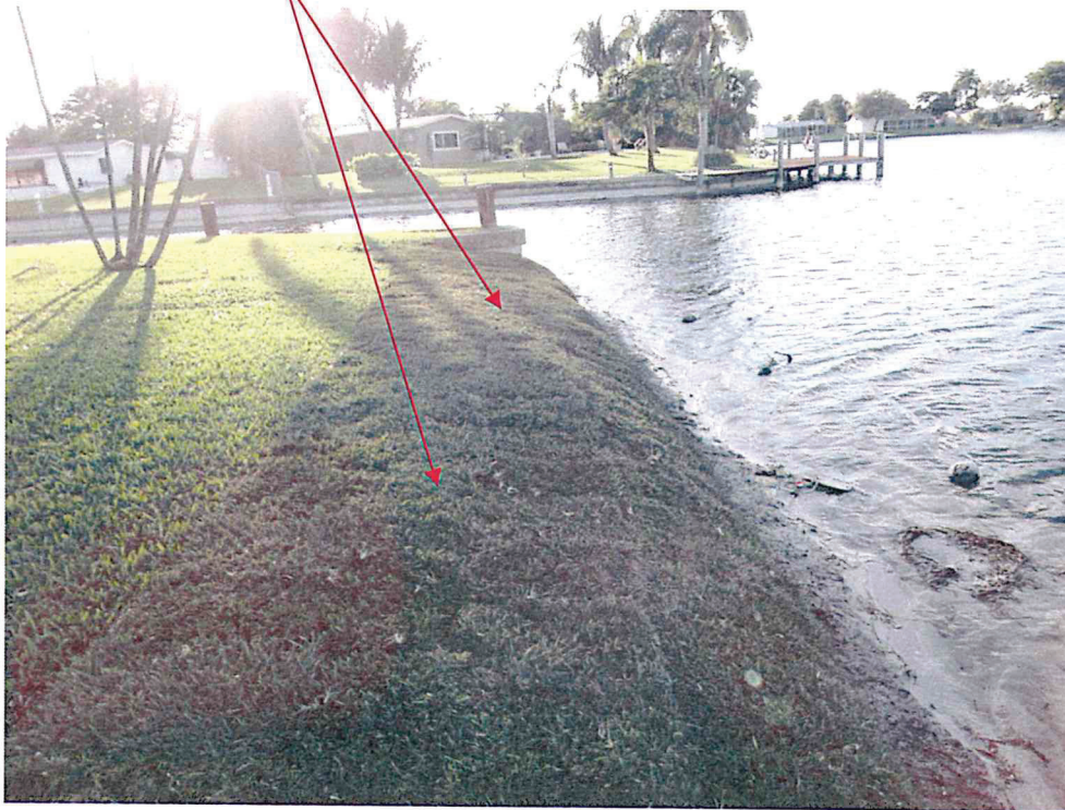
Sod installed over Geo-Tubes and stapled in place
