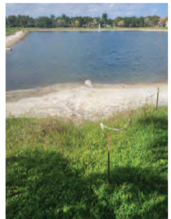
Lake 6 erosion and proximity of drainage culvert between houses
