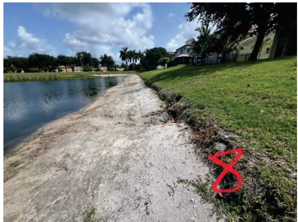
Minor Erosion (8E)
