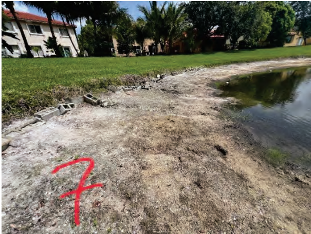
Minor Erosion (7H)
