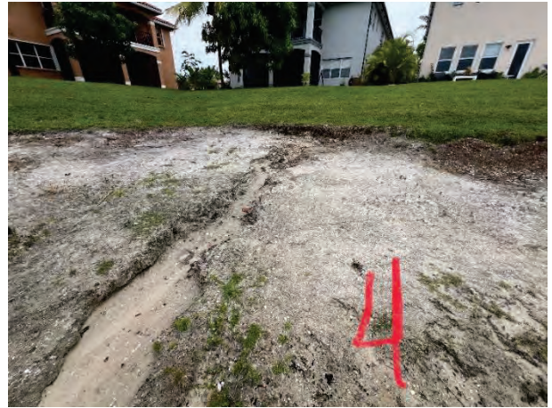
Minor Erosion (4A)
