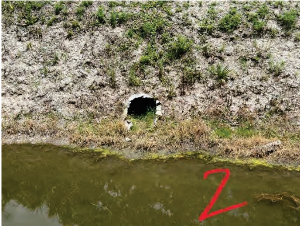
Lake 2 Outfall Leading into LWDD L-4 Canal in Decent Condition
