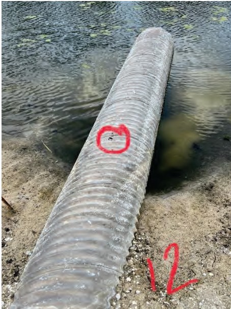
Golf Ball Sized Hole on 24" Outfall (12A)
