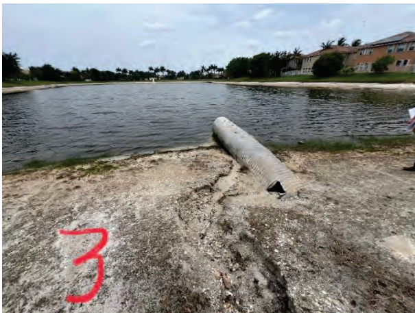
Damaged 30" Outfall (3D)
