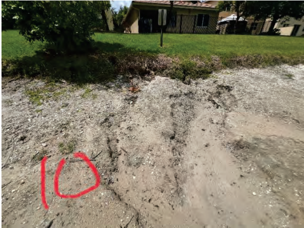
Major Erosion (10F) Bank Beginning to Collapse Pocket Forming Under Bank
