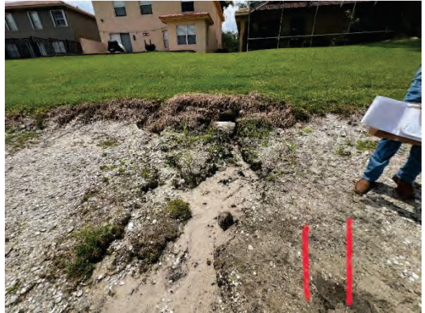
Major Erosion on the East Bank (11G) Pocket Forming Under Bank
