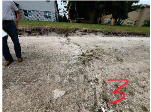
Minor Erosion (3G)
