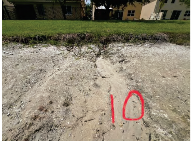
Minor Erosion (10G)
