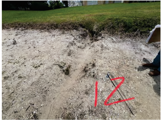
Major Erosion (12E) Pocket Forming Under Bank Bank Beginning to Collapse
