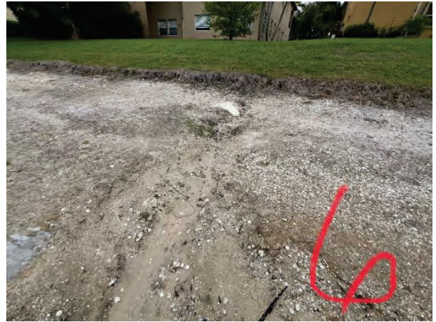
Minor Erosion (6G)
