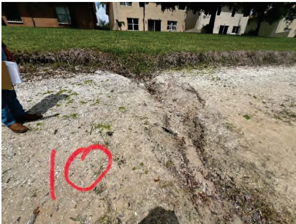
Minor Erosion (10H) Pocket Forming Under Bank
