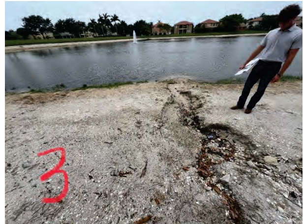
Minor Erosion (3I)
