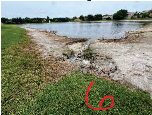
Minor Erosion (6B)
