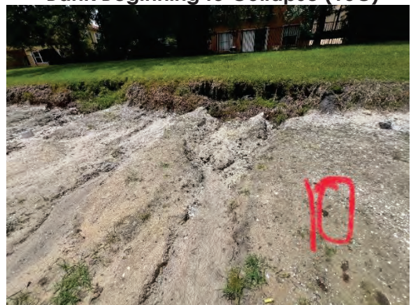
Pocket Forming Under Bank (10E) Bank Beginning to Collapse
