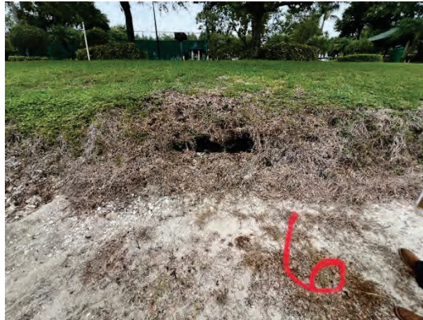
Pocket Forming Under Bank (6H)
