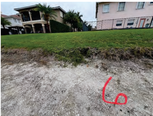
Canal Bank is Beginning to Concave (6D)
