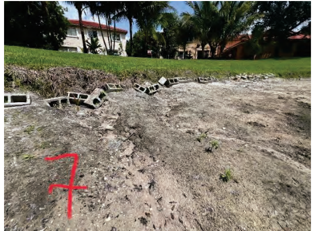
Minor Erosion (7H)
