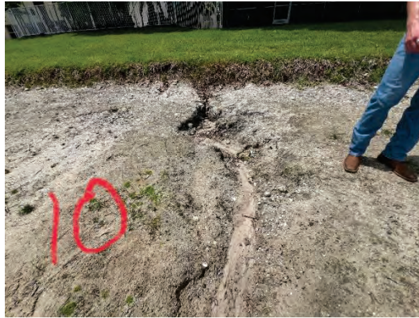
Minor Erosion (10J)
