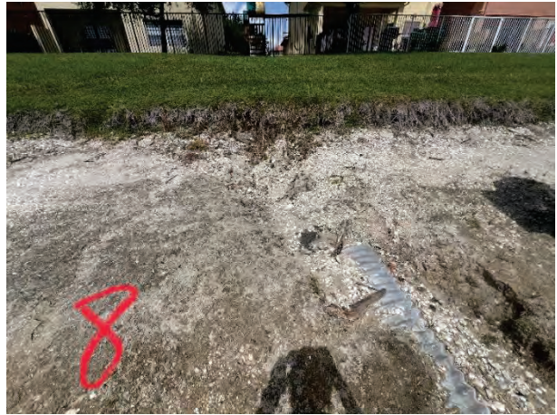
Exposed Outfall Pipe (8K)
