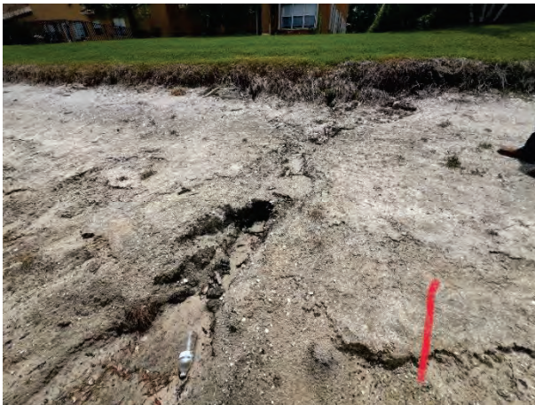
Minor Erosion (1B)
