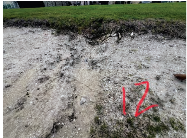
Minor Erosion (12D) Pocket Forming Under Bank Bank Beginning to Collapse
