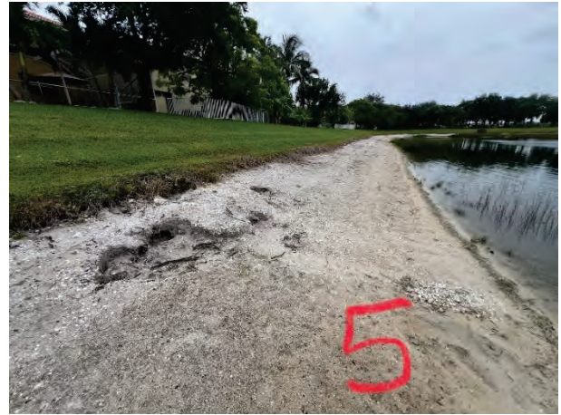
Minor Erosion (5A)
