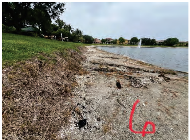
Minor Erosion (6E)
