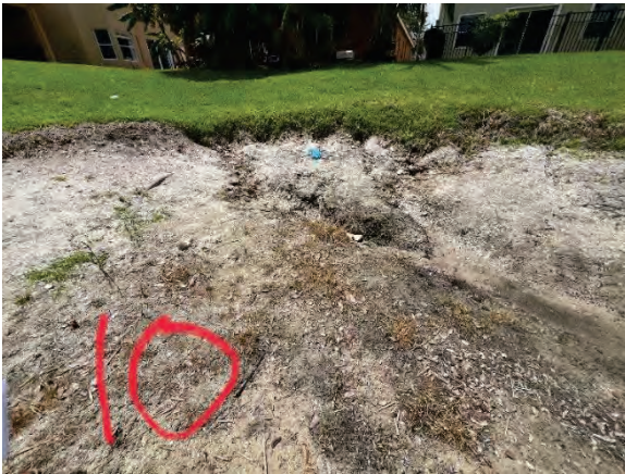
Major Erosion (10B) Pocket Forming Under the Bank
