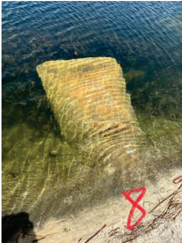
Damaged 30" outfall (8B)
