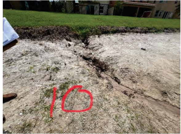
Minor erosion (10A) Pocket Forming Under Bank
