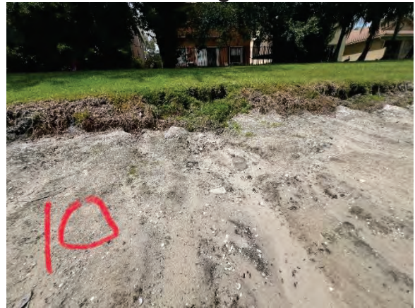
Pocket Forming Under Bank Bank Beginning to Collapse (10C)
