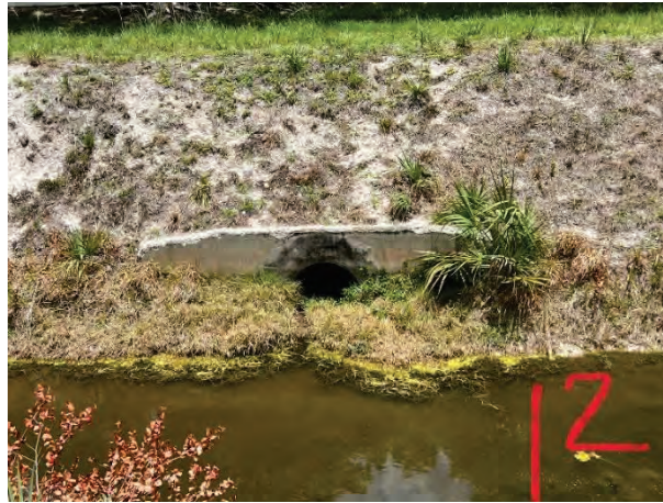
Lake 12 Outfall Leading into LWDD L-4 Canal in Decent Condition
