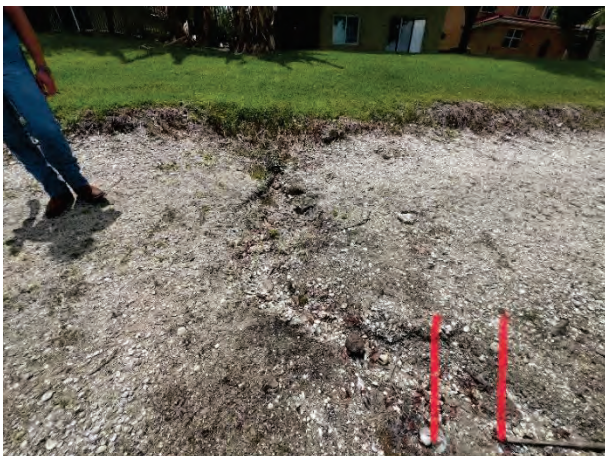
Minor Erosion (11D)
