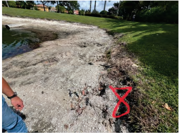
Minor Erosion (8A)
