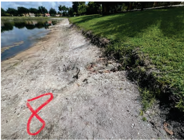
Minor Erosion (8H)
