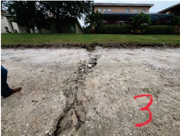
Minor Erosion (3H)
