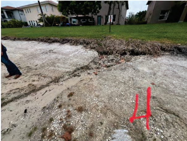
Major Erosion, Grass Caving Down (4B)
