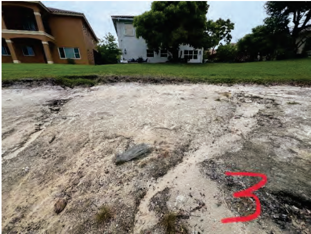
Minor Erosion (3B)
