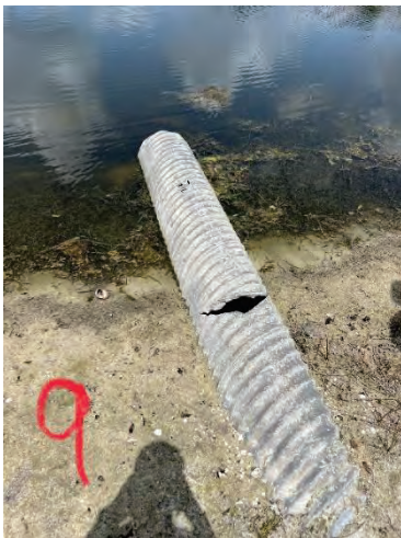
18" Outfall Damaged (9D)
