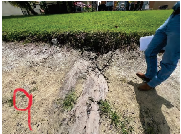
Minor Erosion (9A)
