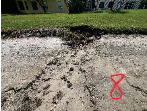
Major Erosion (8F) Lake Bank Concaving
