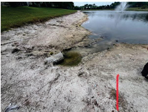
Minor Erosion (1D)
