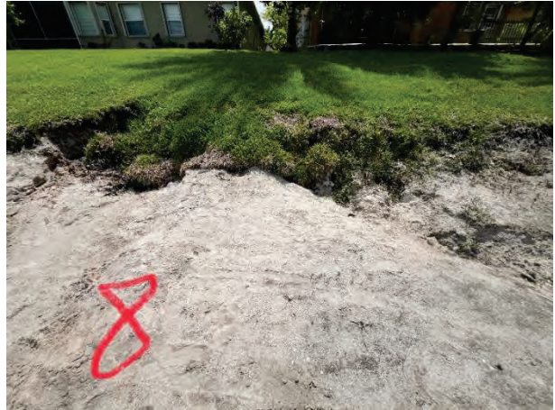
Major Erosion (8G) Lake Bank Concaving
