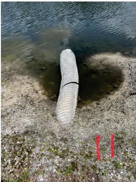
Damaged 18" Outfall (11H)
