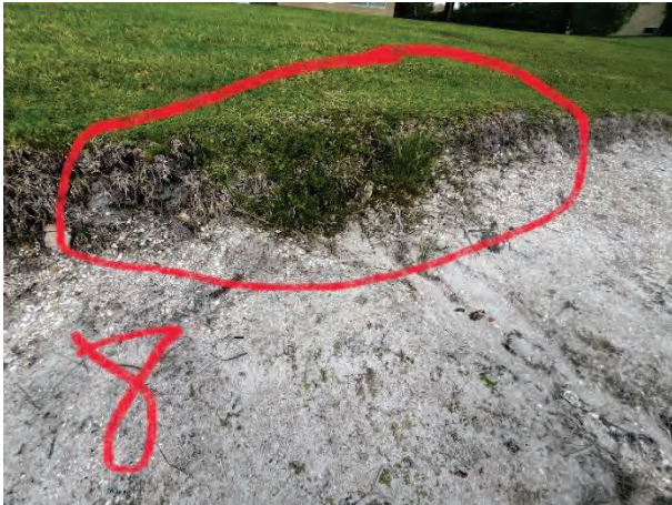
Minor Erosion (8L) Pocket Forming Under Bank
