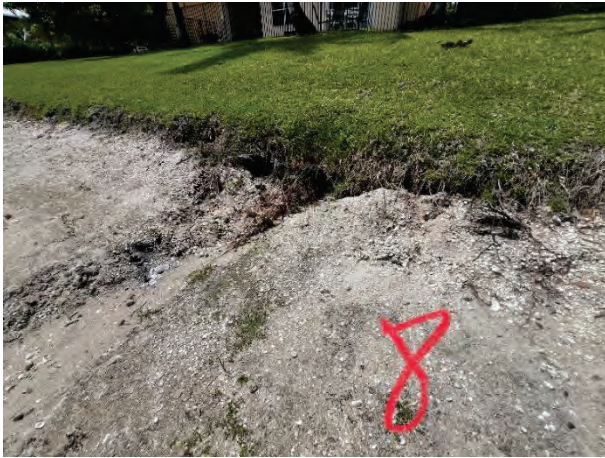
Minor Erosion (8J) Pocket Forming Under Bank
