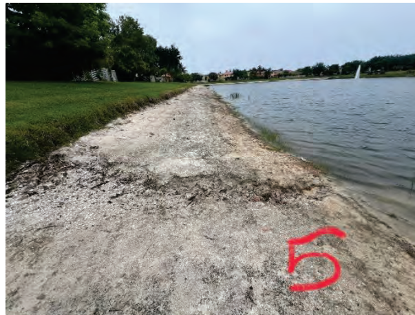
Minor Erosion (5B)
