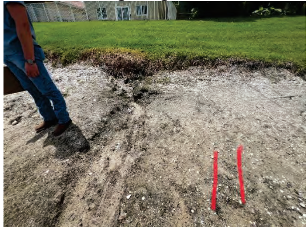
Minor Erosion (11C) Pocket Forming Under Bank
