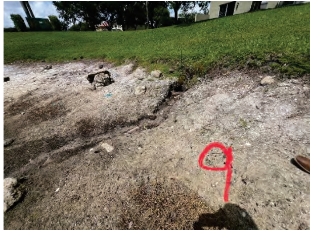
Minor Erosion (9C) Pocket Forming Under Bank
