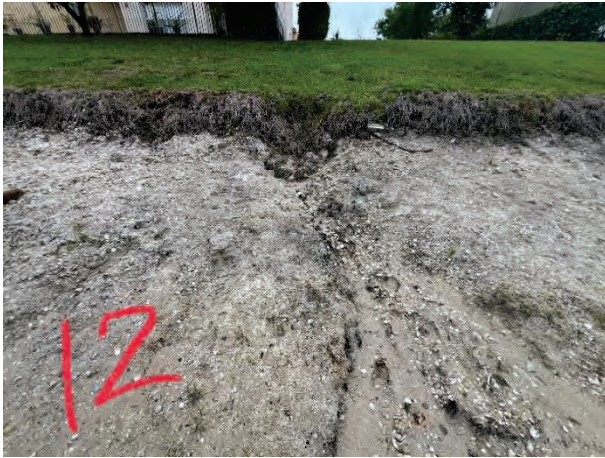
Major Erosion (12D) Pocket Forming Under Bank Bank Beginning to Collapse
