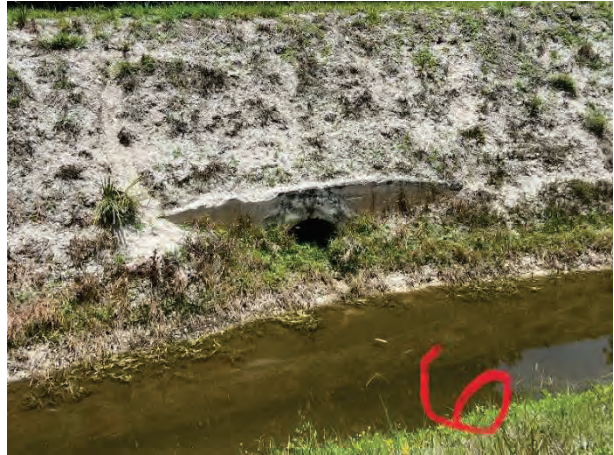
Lake 6 Outfall Leading into LWDD L-4 Canal in Decent Condition
