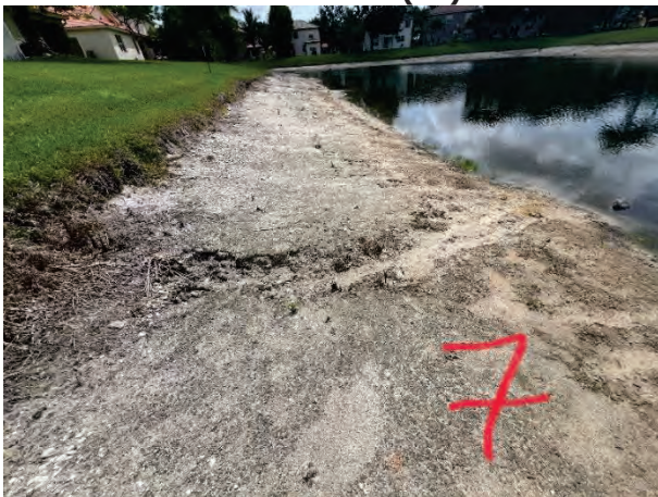
Minor Erosion (7D)
