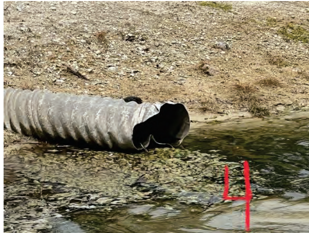
Damaged 30" Outfall (4G)
