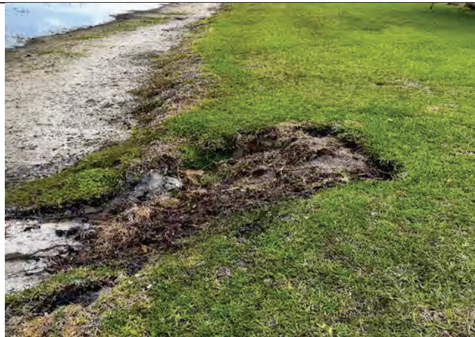
Photo 9: Lake 11 east side north end buried downspout piping
