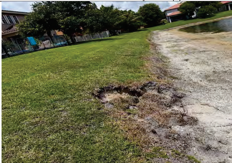
Photo 26: Lake 6 south side by outfall pipe
