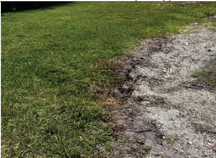
Photo 27: Lake 2 north end of west side
