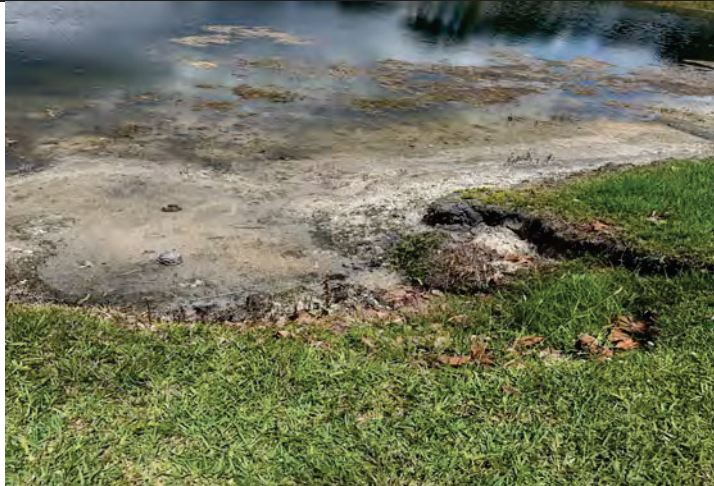
Photo 22: Lake 8 east side
