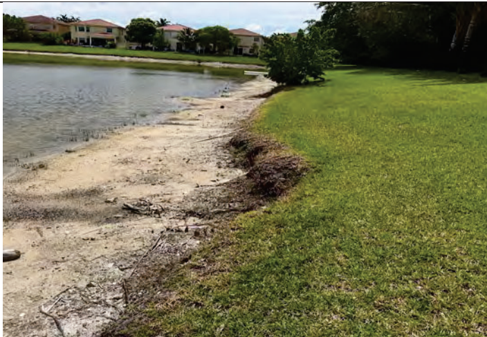
Photo 20: Lake 10 south side west end
