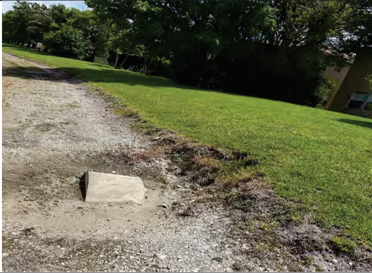
Photo 25: Lake 6 east side by outfall pipe
